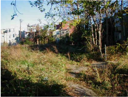
Photo 1: Broken concrete walk
