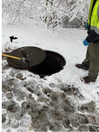
Manhole at 305 Wilmslow Rd located
