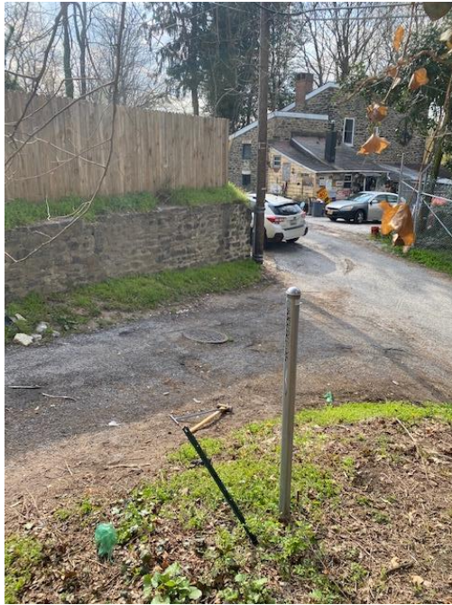
Manhole at 203 Longwood Rd
