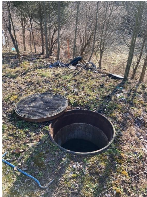
Manhole at 5051 Truesdale Ave uncovered.
