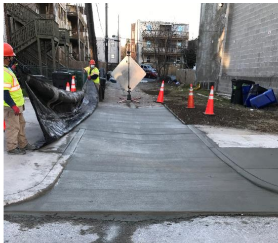
Alley, sidewalk, and curb restoration at 2400 Lakeview Avenue.
