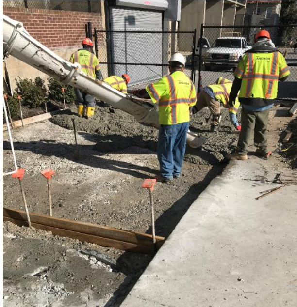
Crew working on concrete restoration at the alley of 2245 Lakeview Avenue
