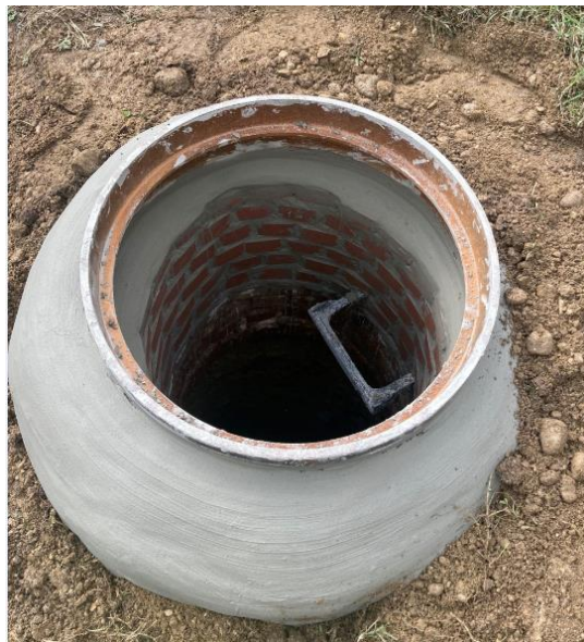
Manhole at located at 4500 Greenspring Ave.
