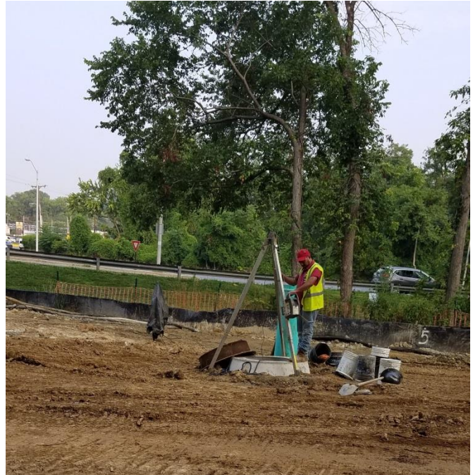
Parging Pipe Joints at Manhole
