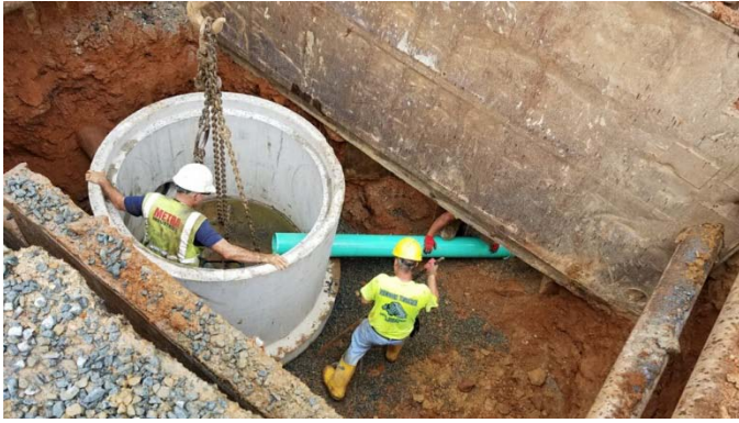
8 in sewer at MH 26
