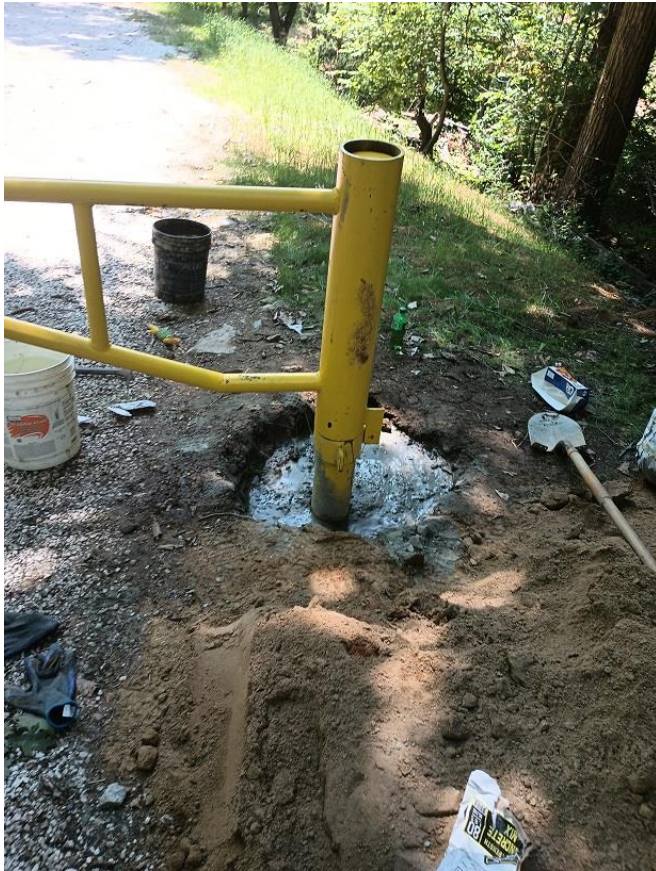
Gate Installation in Leakin Park
