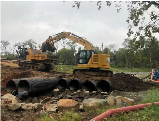
Removing access road and culvert at sta 106+50
