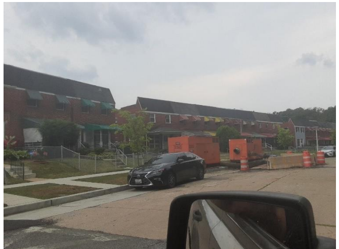
Parking restriction on Kennison (Bypass pumps)
