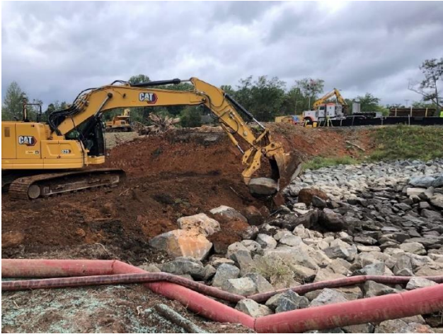
Placing rock at Plunge Pool at sta 106+50
