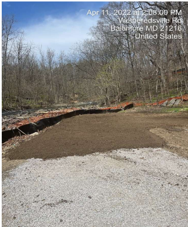
Installation of Geogrid for Access Road
