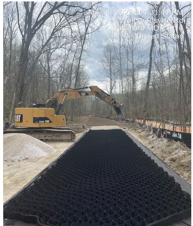
Geogrid being filled in with Stone
