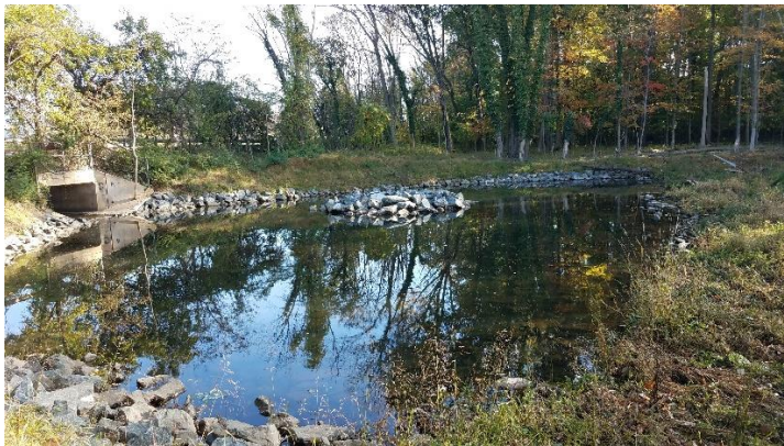
Plunge Pool near Culvert
