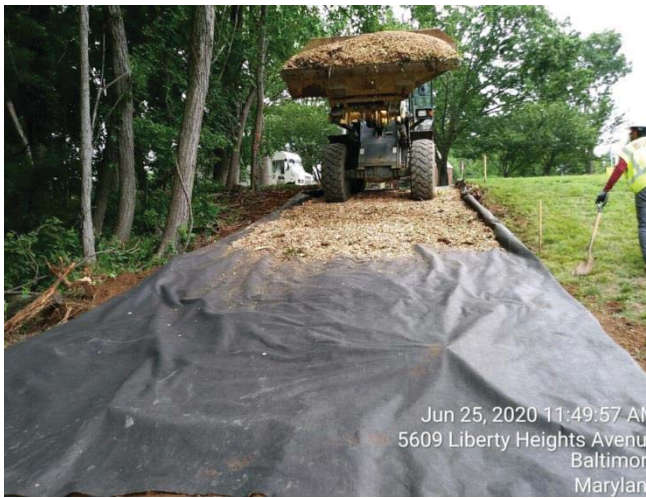
Installing Mulch Matting
