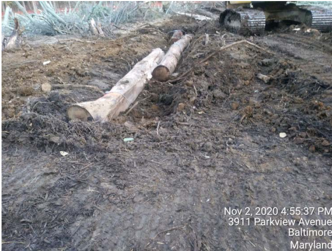
Installing Logs for Stream Restoration
