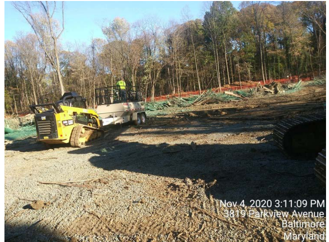
Hydroseed Application in Stream Floodplain
