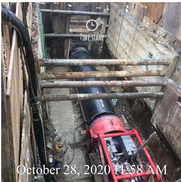
Jacking Pit for Tunnel under Liberty Rd
