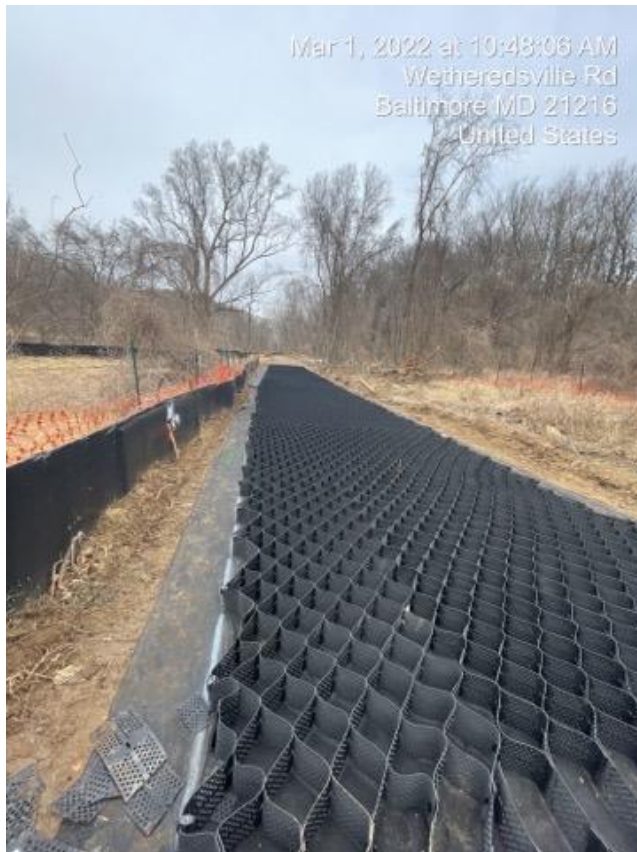
Installation of Geogrid for Access Road
