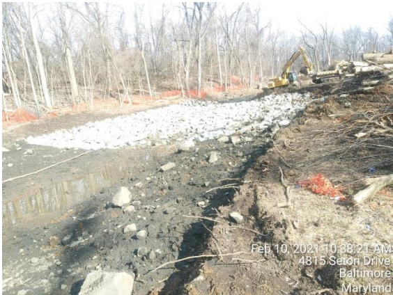
Riprap Installation
