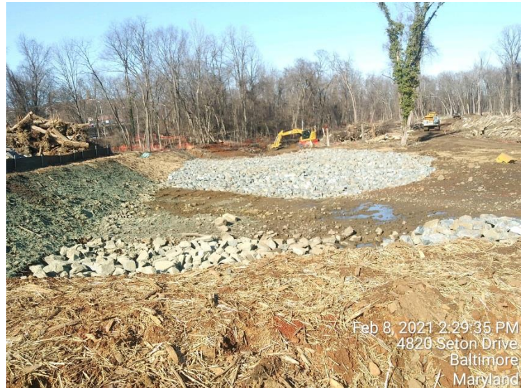
Riprap Installation
