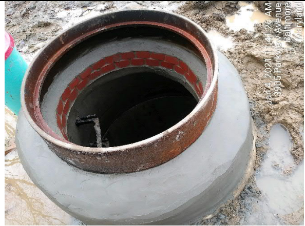
New Manhole Installation
