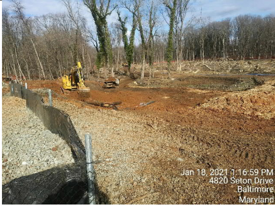
Stream Restoration – Filling Old Stream Bed
