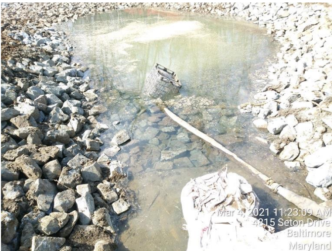
Slope Stabilized with Riprap
