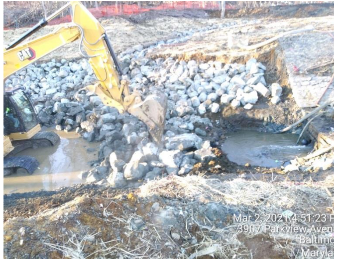
Placing Class II riprap
