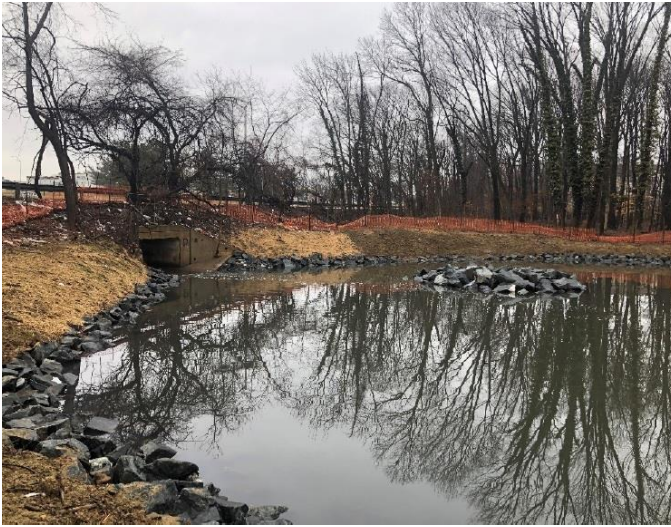
Pool at Culvert Outfall
