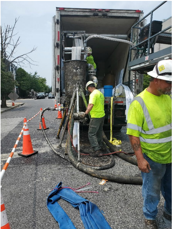
CIPP Liner Installation (E 24 th St)
