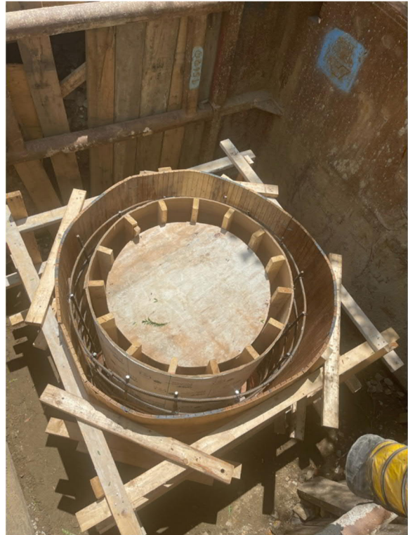
Manhole Seal Application (Falls Rd)
