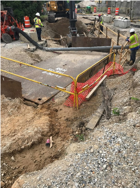
Excavation Backfill (N Broadway)
