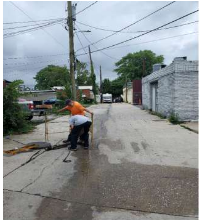
Lateral Cleaning (Camp St)
