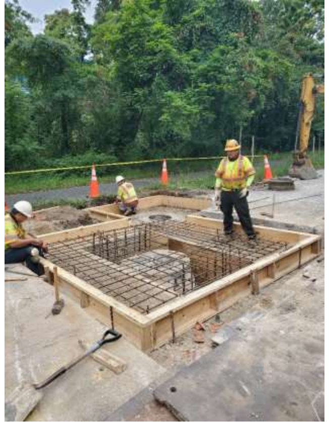
Manhole Seal Application (Falls Rd)
