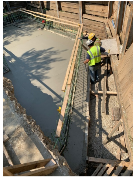
Bottom slab for Structure B poured
