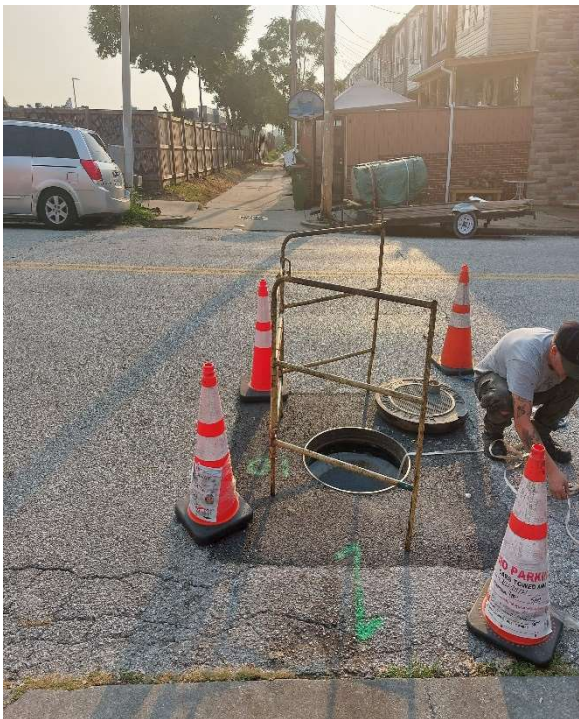
Lateral Lining, CIPP (E 29 th St)
