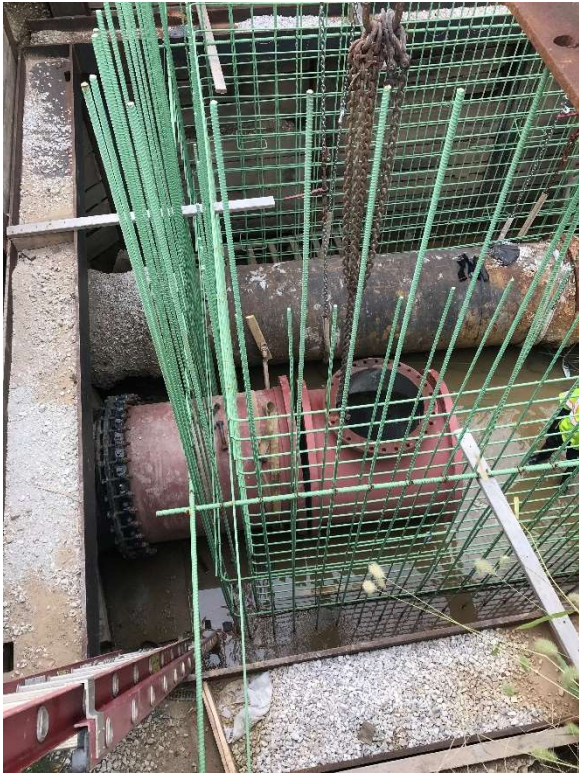
Pressure Sewer (N Broadway)
