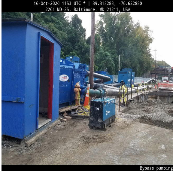
Falls Rd Bypass Pumping
