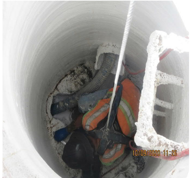
Manhole Rehabilitation – Channel Lining
