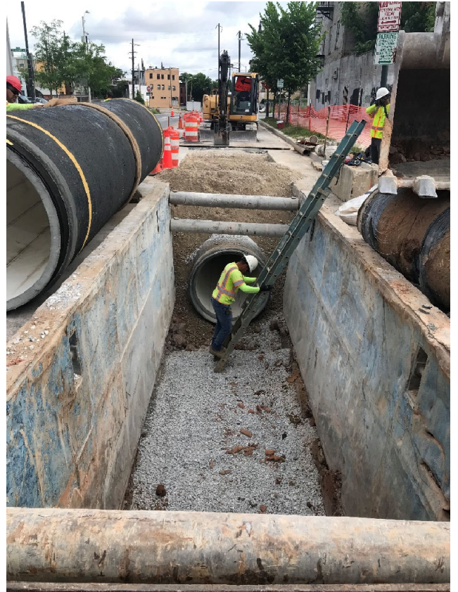
Rutland Ave, PCCP Installation
