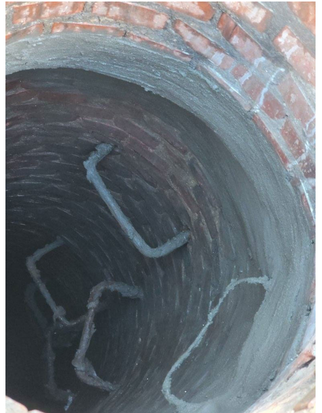
Maryland Ave and Lafayette, Manhole Rehab
