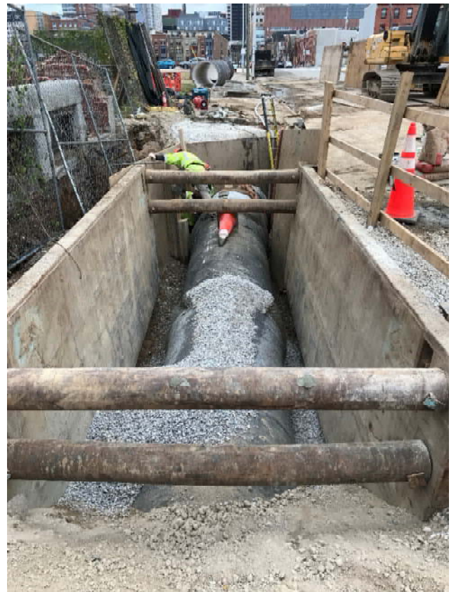
Pressure Pipe Backfill, Rutland Ave
