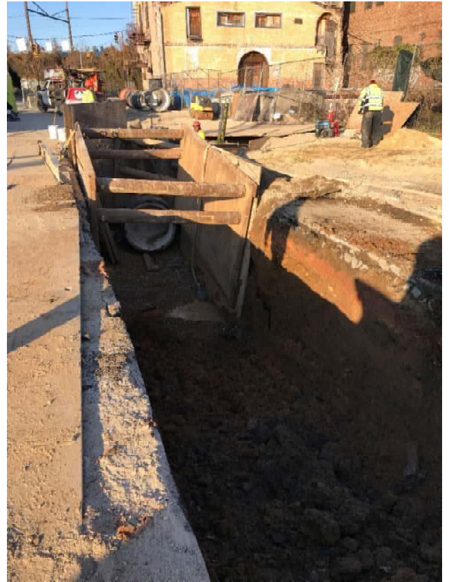
Pressure Sewer Excavation, Rutland Ave
