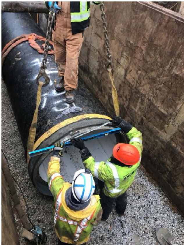
Pressure Pipe Installation, Rutland Ave
