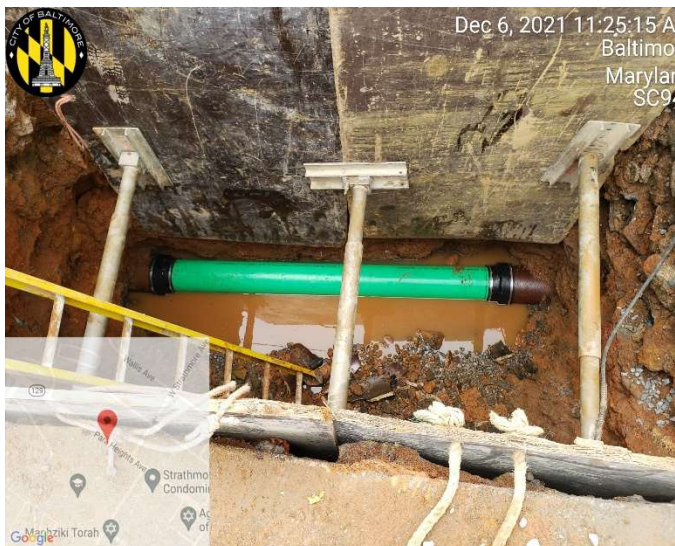
Sewer Rehab (Park Heights Ave)
