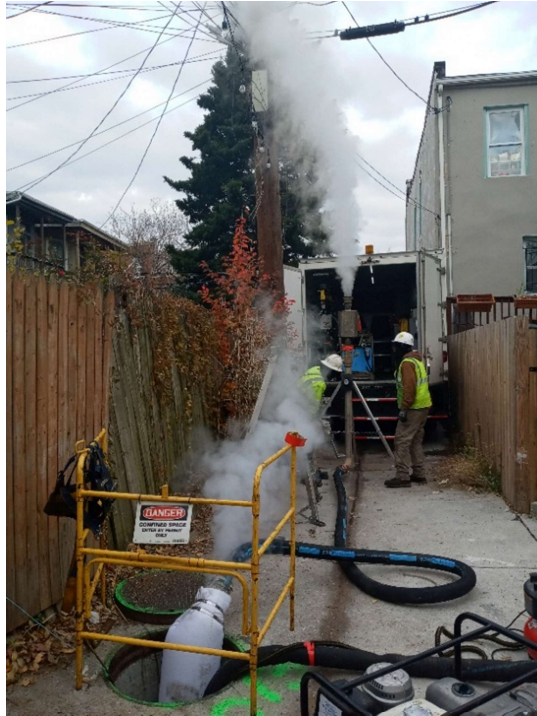
CIPP Lining (Lorraine St)
