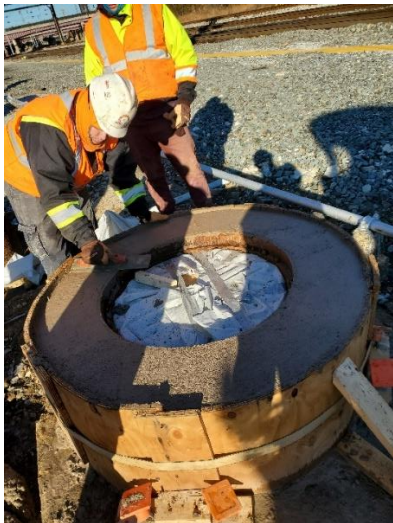
Manhole Rehab (Amtrak-ROW)
