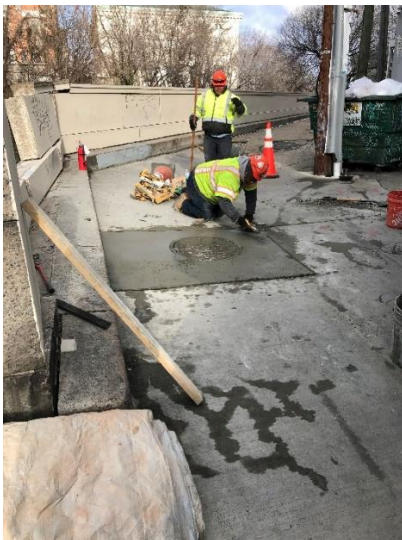
Manhole Rehab (W Biddle St)
