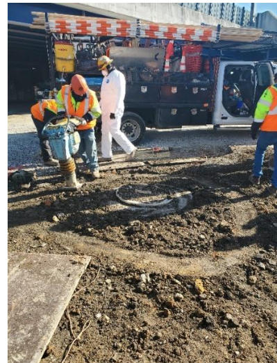
Manhole Rehab (Amtrak-ROW)
