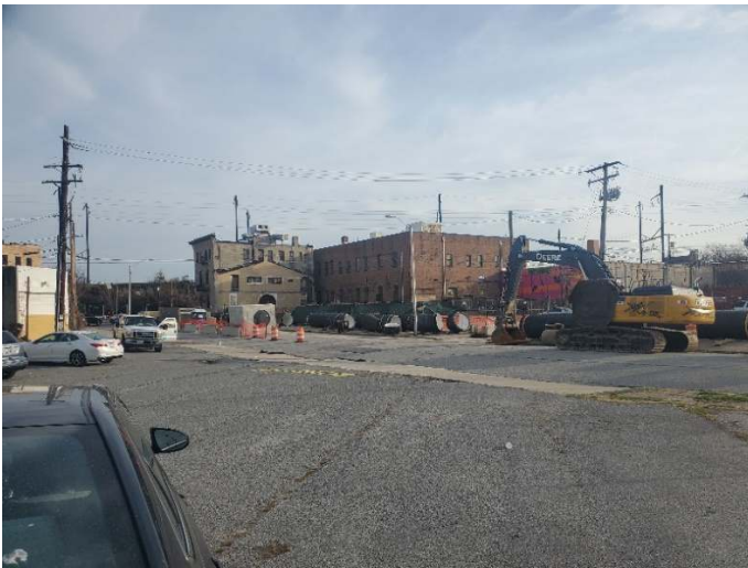
Pressure Pipe Staging (Rutland Ave)
