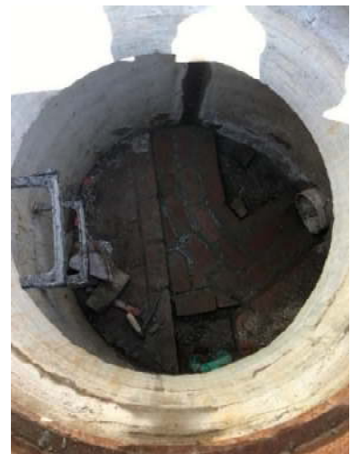
Manhole Rehab (Falls Rd)
