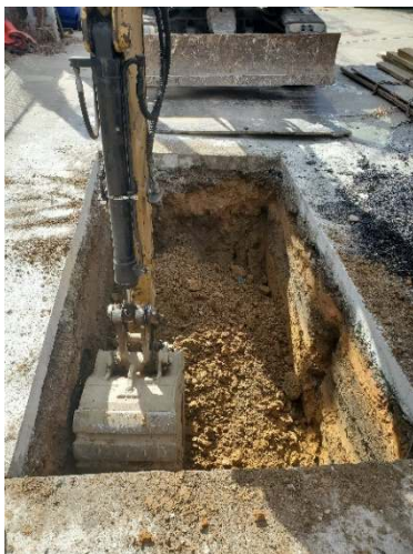
Point Repair (Hunter St)
