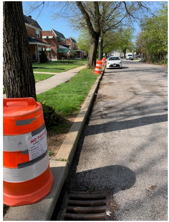
Road Closure Preparation (Midheights Rd)
