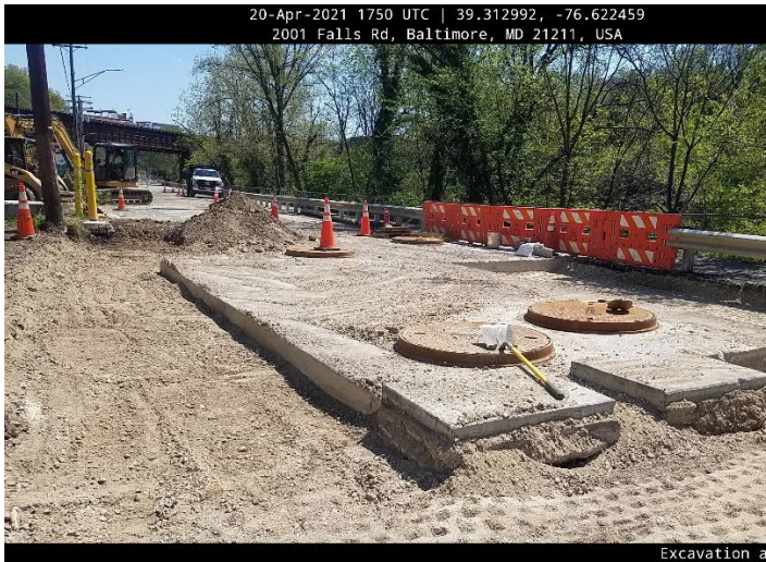
Pavement Restoration (Falls Rd)
