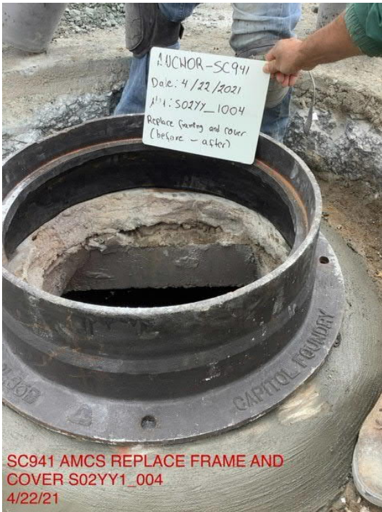
Manhole Rehab (Park Heights)
