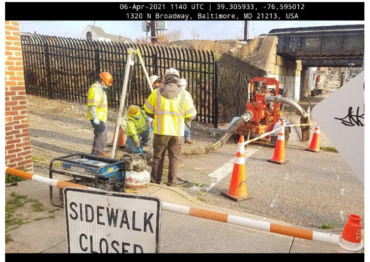
Bypass Pumping Preparation (N Broadway)
