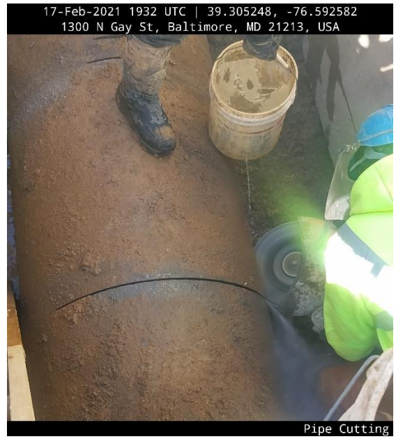
30" Pipe Cutting for Lining Access (Gay St)
