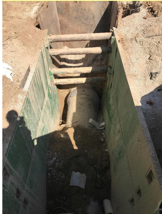
Grout Wrap (N Broadway)
