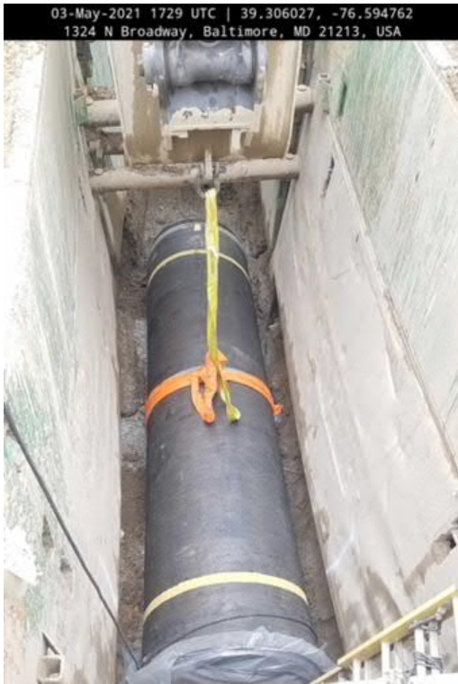
Pipe Replacement (N Broadway)
