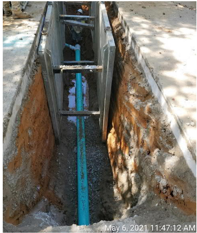
Post Pipe Replacement, (Midheights Rd)
