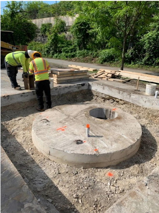
Manhole Seal Prep (Falls Rd)
