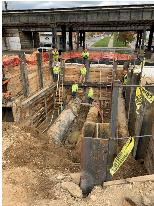
Excavation for Vault 1 (Broadway)
