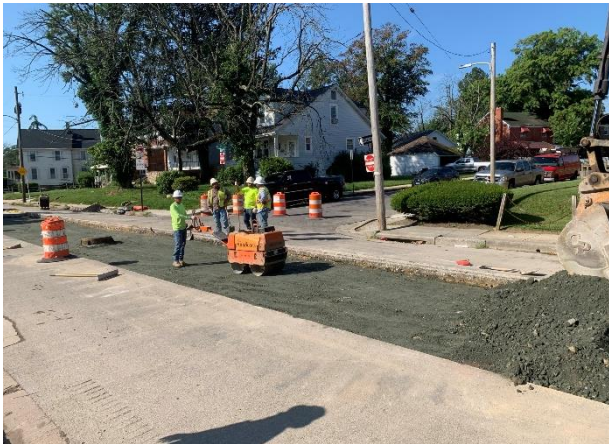
Concrete roadway restoration along 3900-4000 Block of Callaway Avenue
