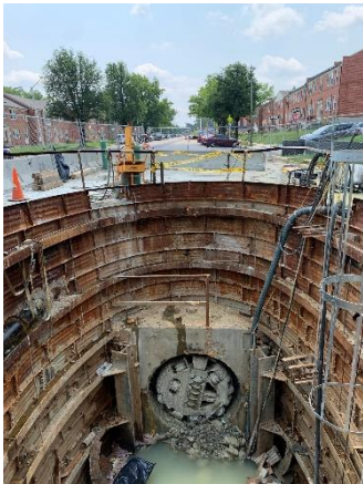
Microtunnel machine breakthrough at 3910 Wabash Ave (segment completion)
