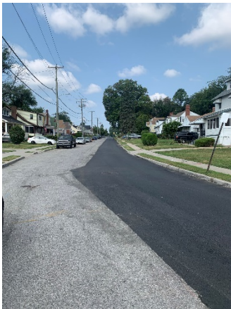
Asphalt roadway repairs in-progress at 3700-3800 W Cold Spring Lane
