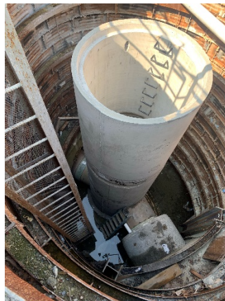
Manhole construction underway at Liberty Heights Avenue & Wabash Avenue
