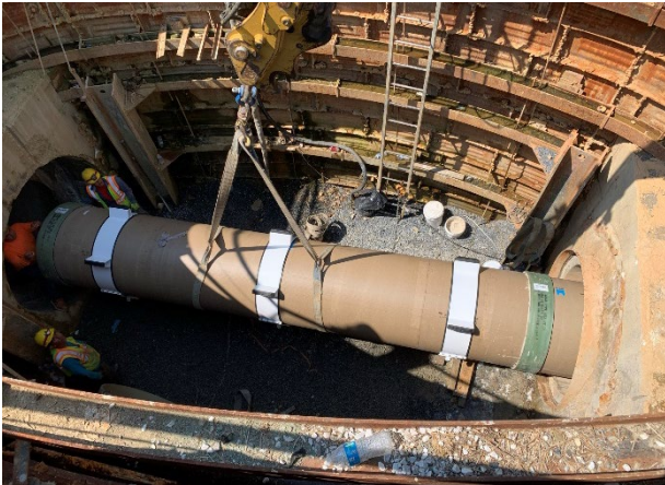
42" GRP slip-lining in-progress at The 3900 Block of Wabash Avenue
