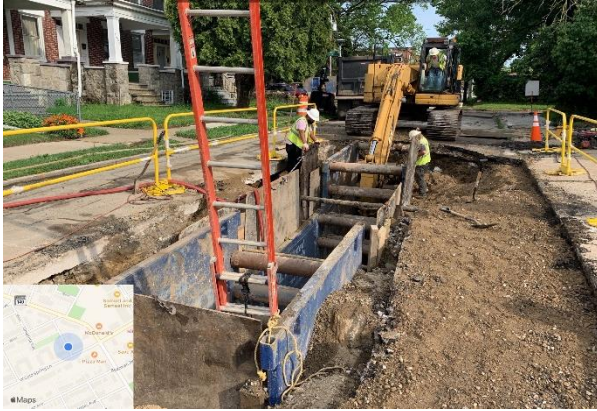
New 30" sewer pipe construction along Towanda Avenue approaching Ridgewood Ave
