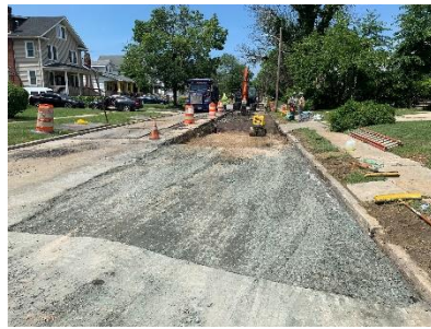
Open-cut sewer upsizing replacement underway along 3700 block of Belle Ave
