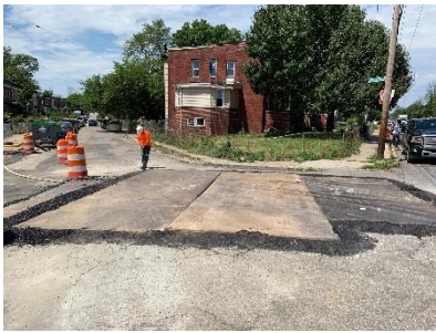
Open-cut sewer location at Ridgewood Ave & Reisterstown Road
