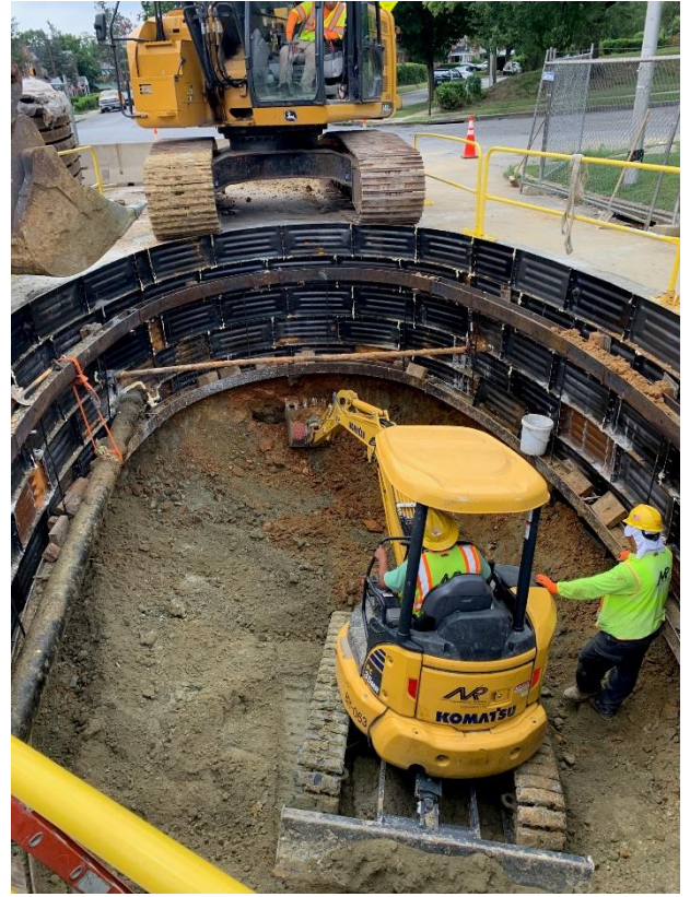
Shaft #6 construction underway at Sequoia Ave & Wabash Ave
