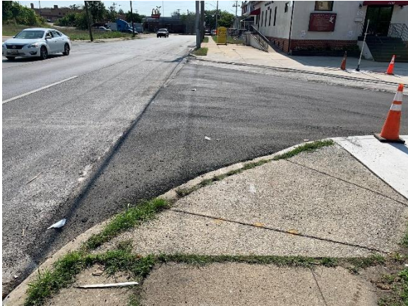
Asphalt paving at Ridgewood Ave. & Reisterstown Road (August 2022)
