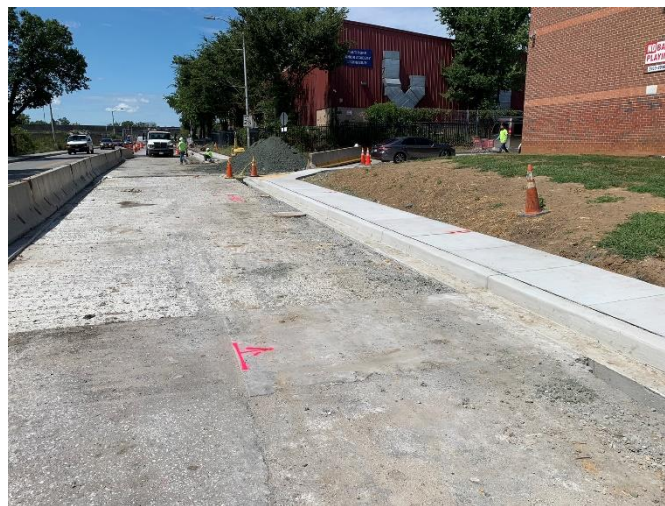
New curbs and sidewalks at 2900 W. Cold Spring Ln. (August 2022)
