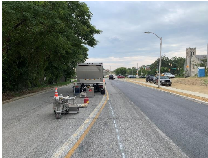
New asphalt and striping (underway) at 2800 N. Dukeland Street (September 2022)
