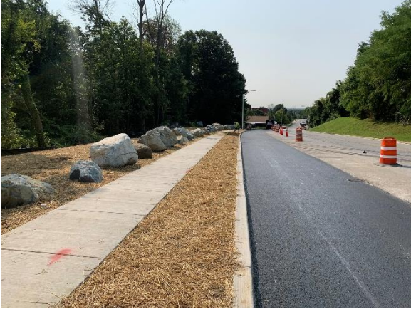
New sidewalks and curbs at 2800 N. Dukeland Street (September 2022)
