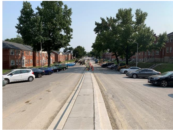
New concrete medians at 4000 Wabash Avenue (August 2022)
