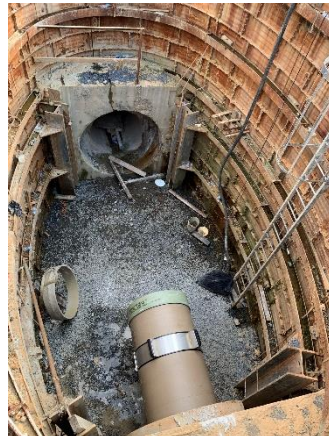
42" GRP slip-lining in-progress at The 3900 Block of Wabash Avenue
