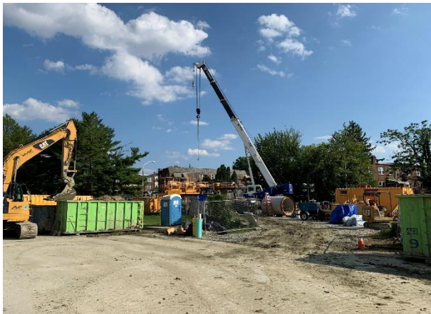
60" microtunneling underway at the MTA lot at Wabash Avenue
