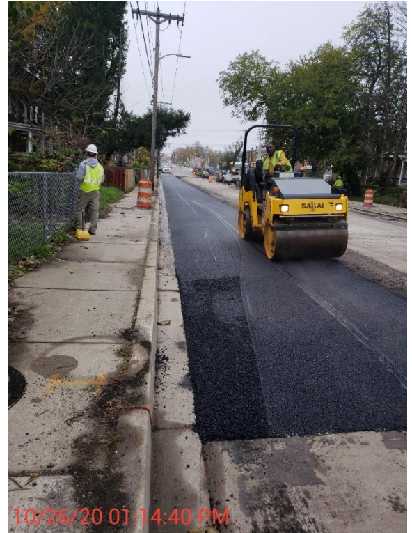
Asphalt paving at 4600 Reisterstown Road
