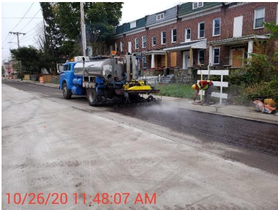
Restoration underway at 4500 Reisterstown Rd
