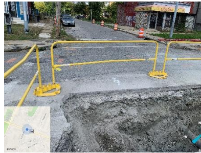
Open-cut excavation work underway at Virginia Ave & Reisterstown Road
