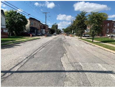
Pipeline work completed along Reisterstown Road, temporary patching in place
