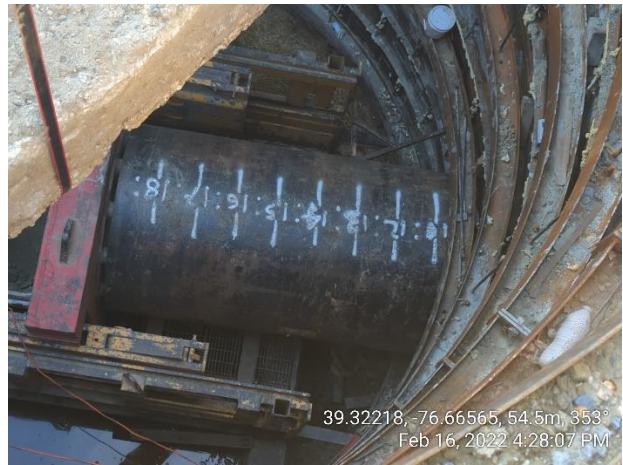
Micro tunneling progress at Dukeland Street under 84" main
