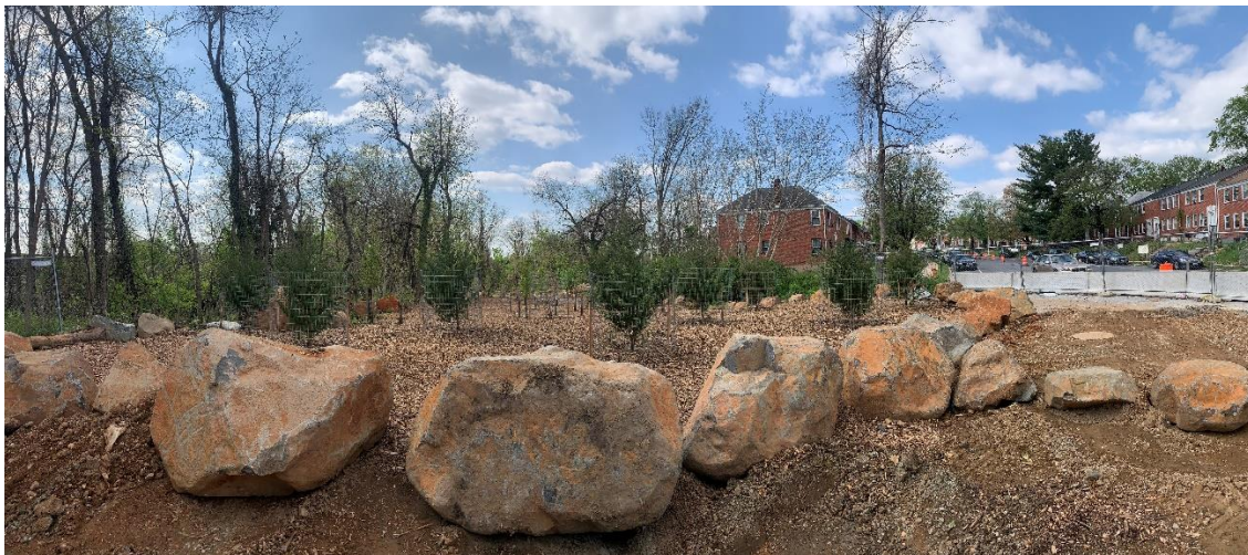
New tree plantings and stone placement at 4000 Block of Hilton Road (Completed April 2022)
