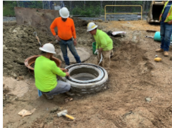
Installation of new 96" manhole at 2800 N. Dukeland Street. (Completed June 2022)
