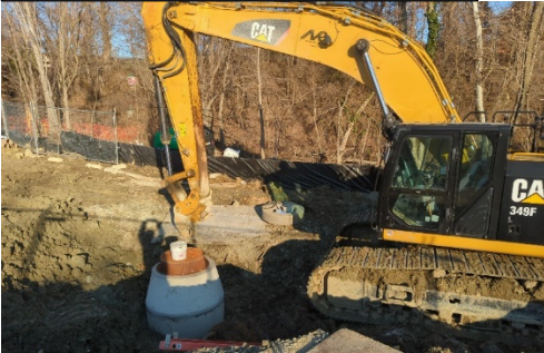
Manhole Installation on Dukeland Street
