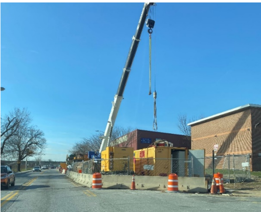
60" microtunneling starting at 3000 blk of W. Coldspring Lane
