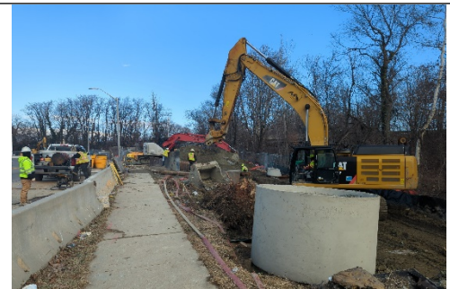
Part of worksite at Dukeland St.
