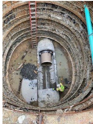
Relief sewer slip-lining at 3500 Blk Wabash Avenue
