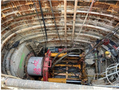
Microtunneling underway at 3801 Wabash Avenue
