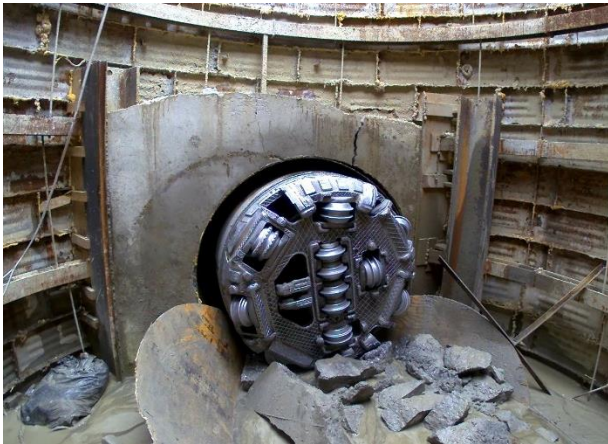
Microtunneling machine exit at completion of tunnel @ 3600 Blk Wabash Ave
