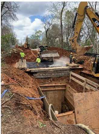
Open-cut casing installation in ROW near Wabash Ave & Hilton Road
