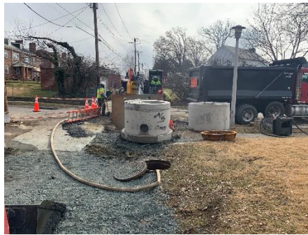
Sewer construction at 3800 Blk Grantley Ave underway
