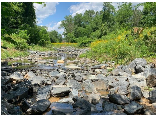
Overlooking completed stream work in Reach F above Belvedere Ave
