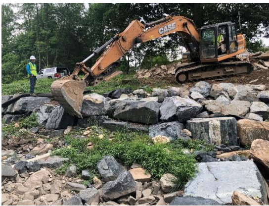
Stream rock wall construction in Reach D
