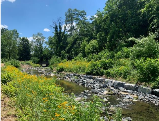
Stream and sewer work completed north of East Belvedere Avenue
