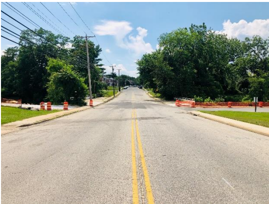
Sewer work at 1270 / 1301 Woodbourne Ave completed and roadway reopened
