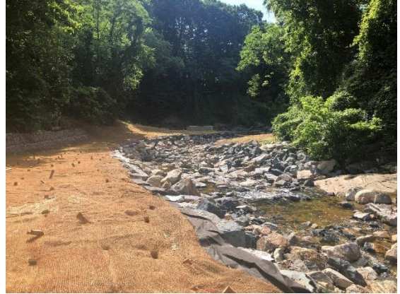
Stream repairs completed East of Hillen Road near Morgan State University
