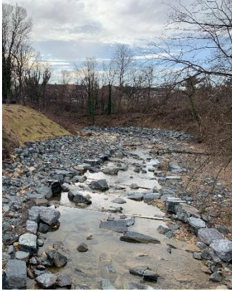
Completed stream restoration work at Woodbourne Avenue
