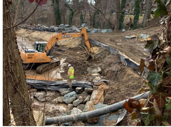
Stream restoration underway between Northern Parkway and East Lake Avenue
