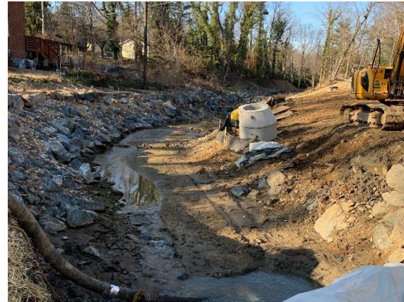
Temporary stream diversion being setup at Chinquapin Run
