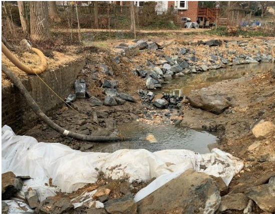
Temporary stream diversion being setup at Chinquapin Run
