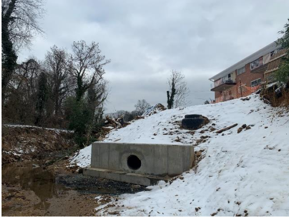
New stormwater headwall installed behind 6200 Chinquapin Parkway & 6200 Northwood Drive
