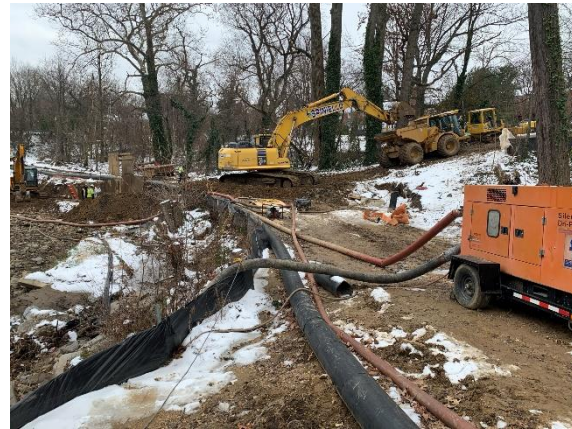
Sewer construction underway between Northern Parkway and E Lake Avenue
