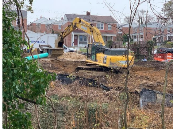
Sewer replacement underway behind 6200 Chinquapin Parkway
