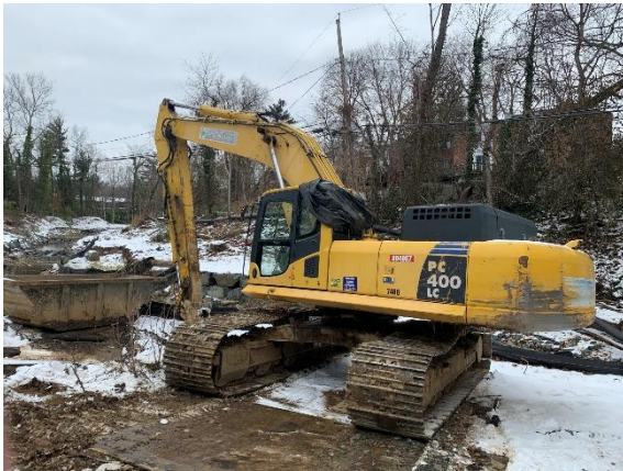
Sewer construction underway above E Lake Avenue @ Chinquapin Run crossing
