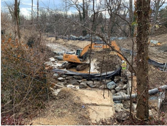
Stream restoration in progress upstream of Northern Parkway
